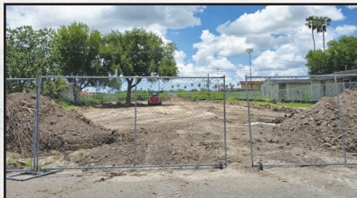
Le Moyne Gardens parking project
