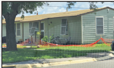
Le Moyne Gardens roofing work
